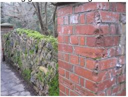
East end: London Clay beneath the weir from Jack's Lake; over-burnt bricks on the bridge over Pymms Brook coming from Jack's Lake – an indication of local brickmaking probably from the silty Claygate beds.
